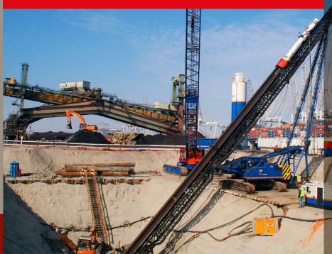
When it comes to installing foundations and quay walls for complex maritime projects, steel structures are the best solution. As a result of its unique design, the Hydrohammer® is perfectly suited to driving steel piles and essential for a successful installation. To handle these hammers, specialised piling rigs are required, for which IHC IQIP is the supplier of the world's largest piling cranes.
